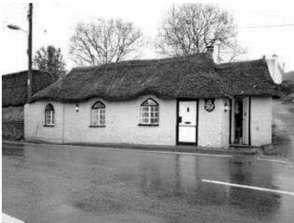
Illustration 5. Toll House in Newton Poppleford in Sidmouth, Devon
