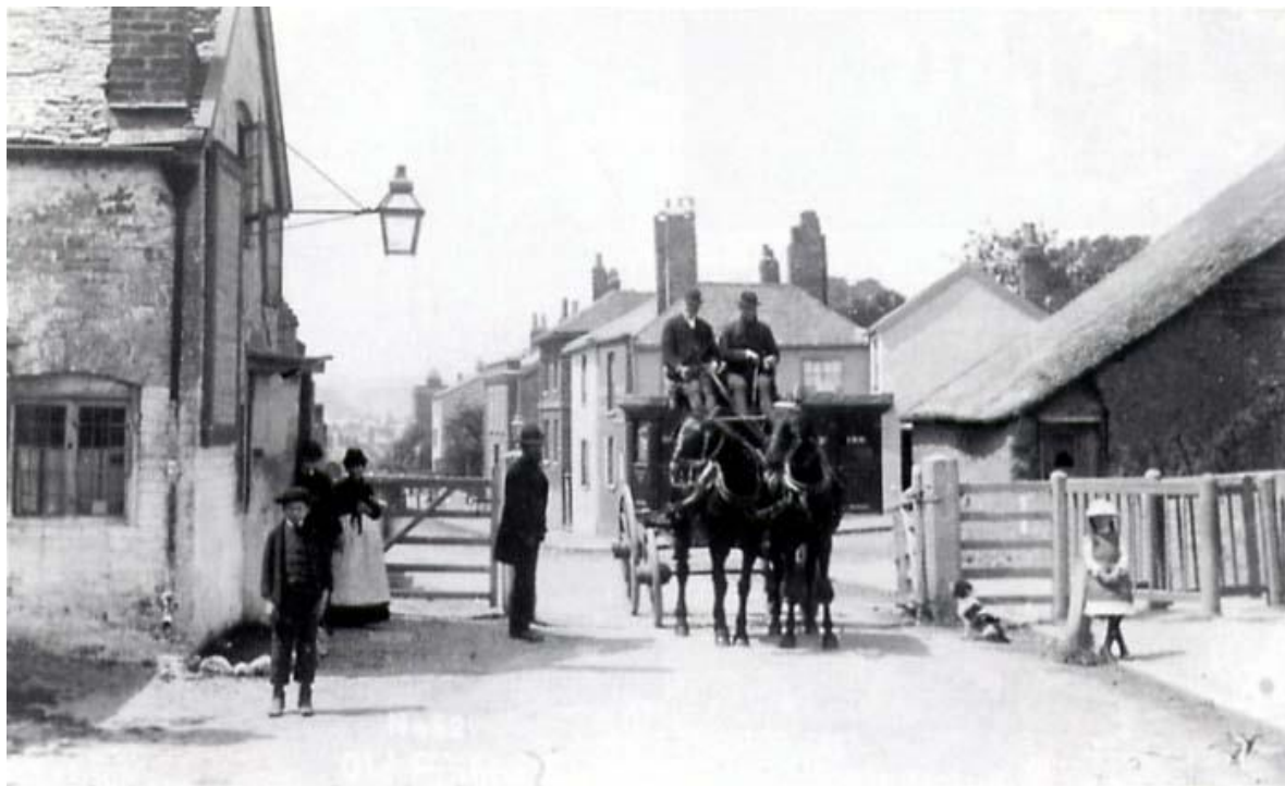
Illustration 4. Toll House at the junction of Blackboy Road & Mount Pleasant Road, circa. 1884 in Heavitree
